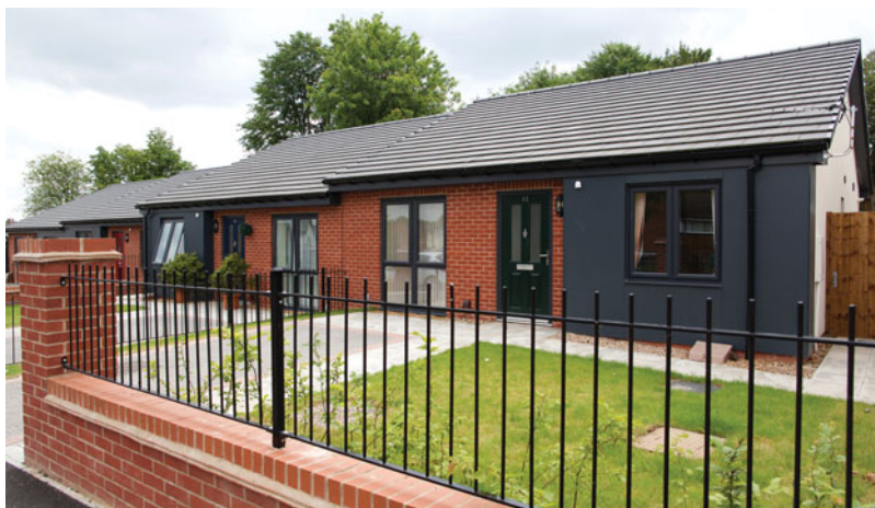
Nottingham City Homes, Cranwell Bungalows, a development of 11 bungalows
